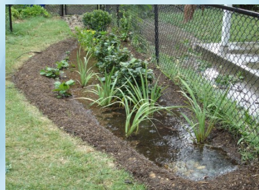
Plantings in the basin must be able to withstand periods of inundation
