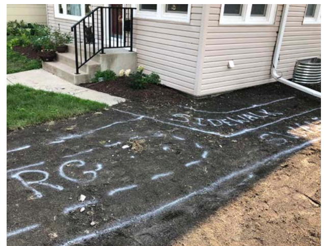
Raingarden basin sited the proper distance from a house
