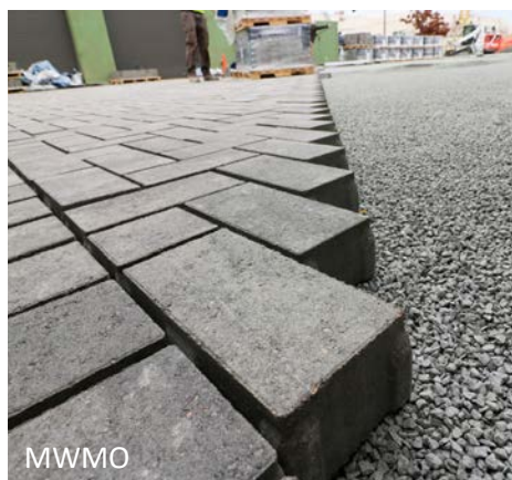
Permeable pavers with bedding course
